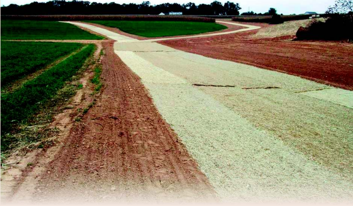
Newly constructed grass waterway
